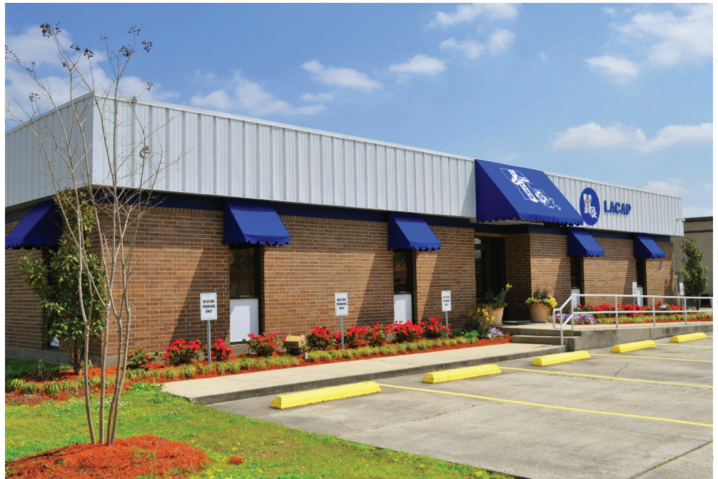
The LACAP Weatherization Training Center provides 17,000 square feet of classroom, office, lab and state-of-the-art demonstration and hands-on training modules space.
